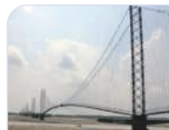
Dodhara Chandani Longest Suspension Bridge
